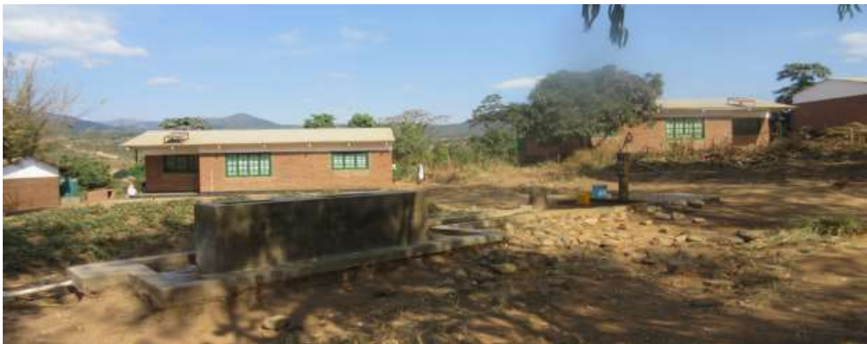
FIGURE 5 TEACHERS’ HOUSING KAYELEKERA PRIMARY SCHOOL, BOREHOLE AND SOLAR PANELS
