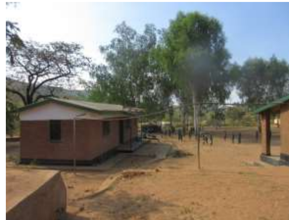
Kayelekera Primary School showing Solar Power system provided by Paladin
