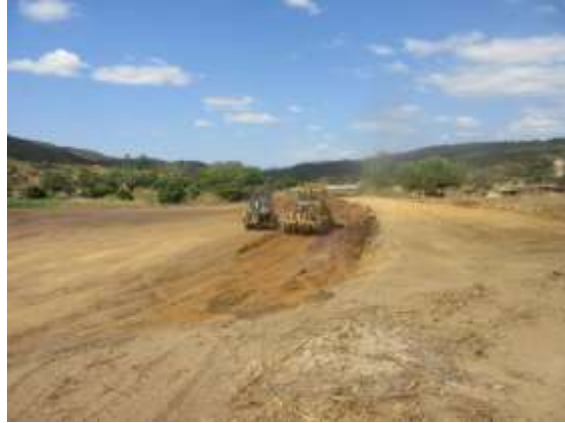
Grading for the clinic in Kayelekera, June 2015
