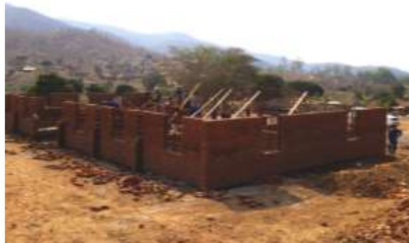
Progress - Kayelekera Clinic - Sept 2015
