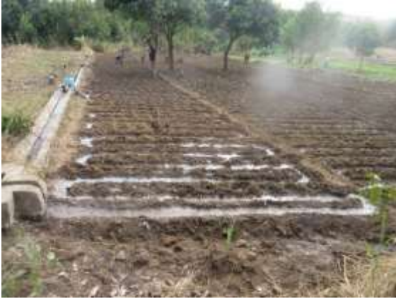
Successful Irrigation System provided by the Mine now used by farmers coop
